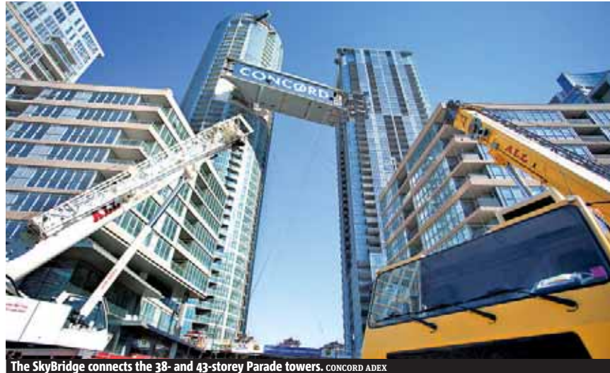
The SkyBridge connects the 38- and 43-storey Parade towers. CONCORD ADEX
