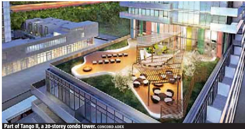
Part of Tango II, a 20-storey condo tower. CONCORD ADEX
