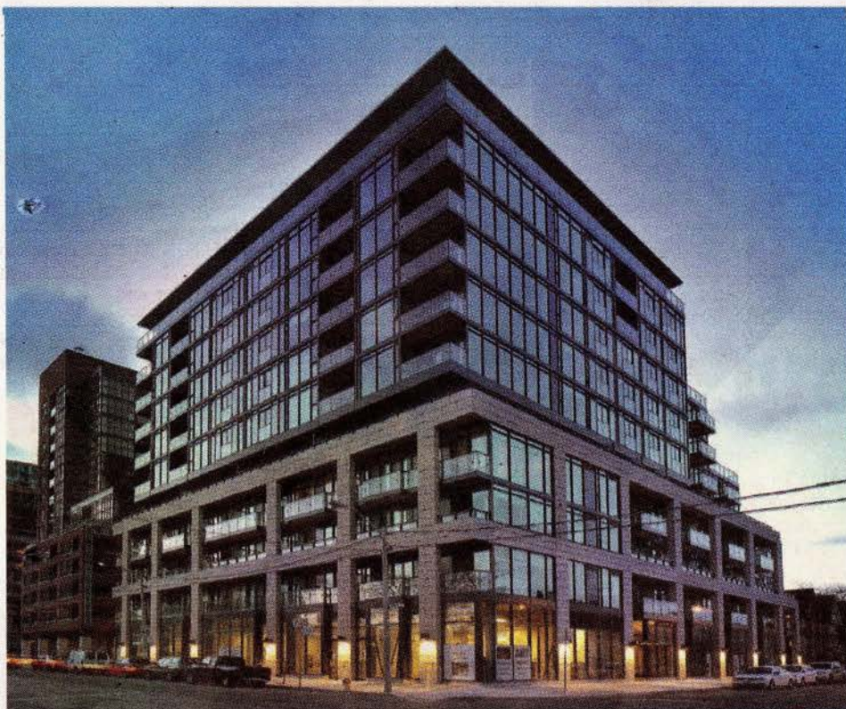
ART condominiums is a unique 11-storey, terraced mid-rise located in the heart of the Queen West arts community.
